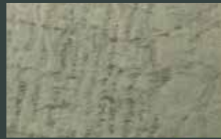
6362ST 6 Concrete Formwood
